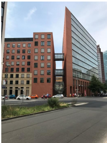
Figure 16. The Building Material "Terracotta" Used in Facades (Author's archive, 2020)
